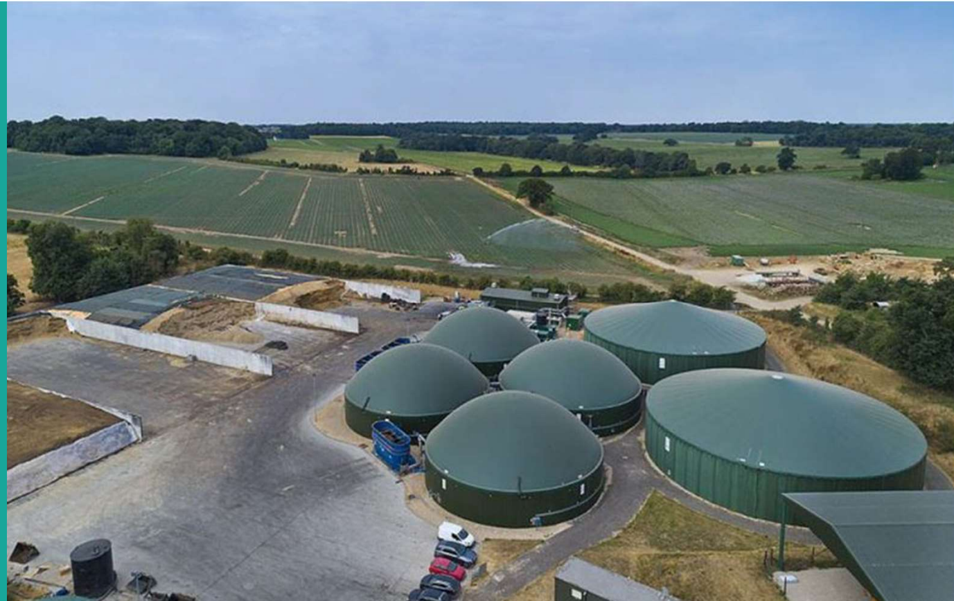
The Euston Biogas Plant, located near Thetford, Suffolk Image courtesy of Material Change
